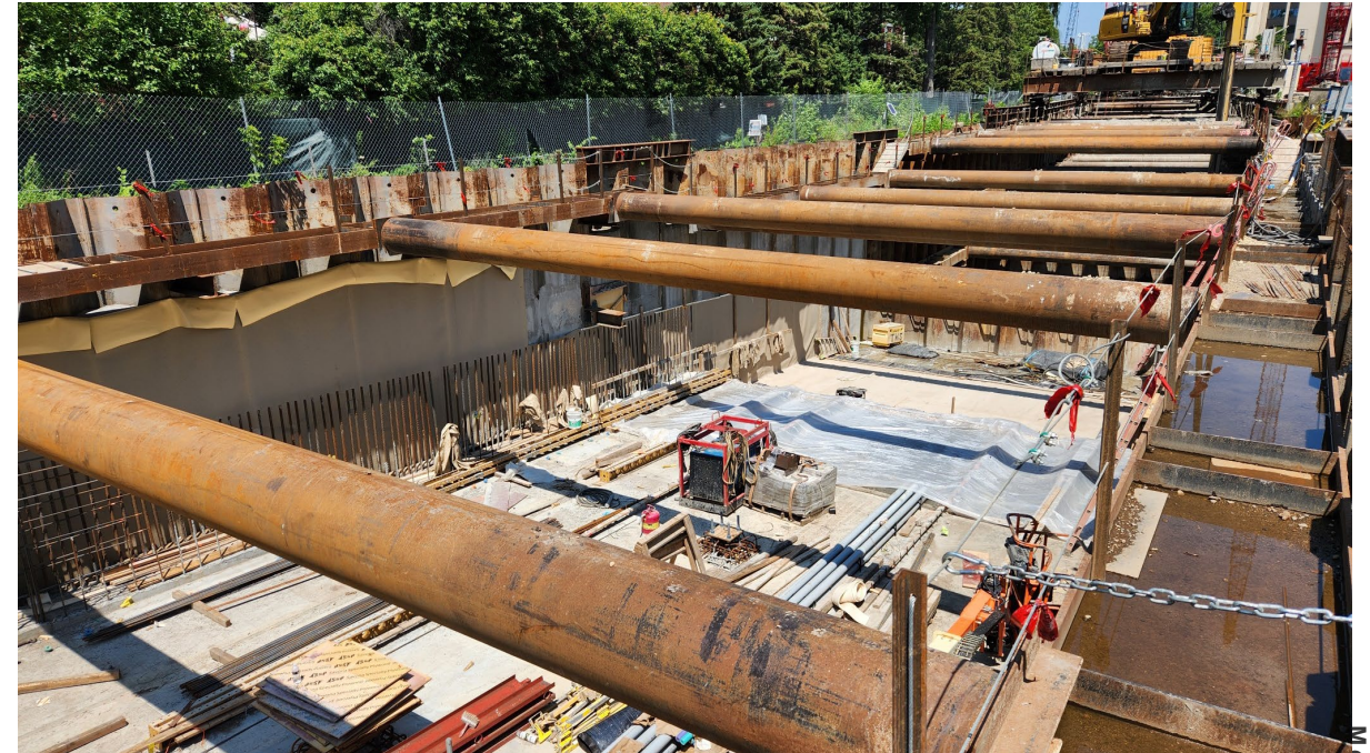
Kenilworth LRT tunnel: waterproofing installation
