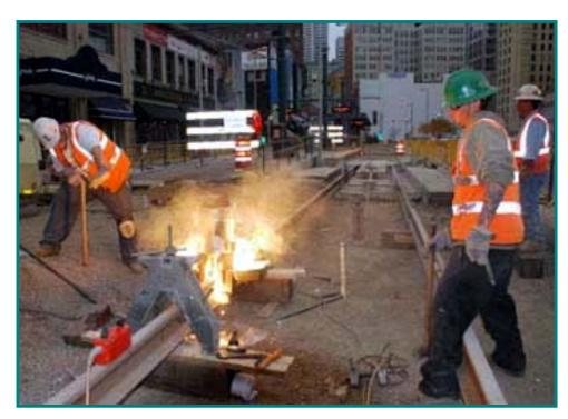
Welders Britton Carpenter and Brian Downey of Chesapeake Thermite Welding finished the final welds in the Hiawatha LRT extension on November 5.
