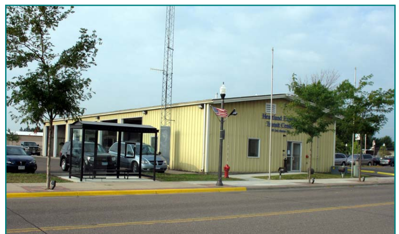
Newly remodeled Chisago County Heartland Express Transit Center
