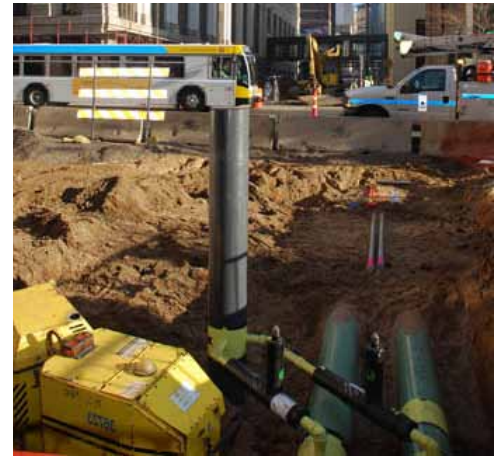
Relocation of utilities in downtown St. Paul, in preparation for construction of Central Corridor LRT, began in 2009.
