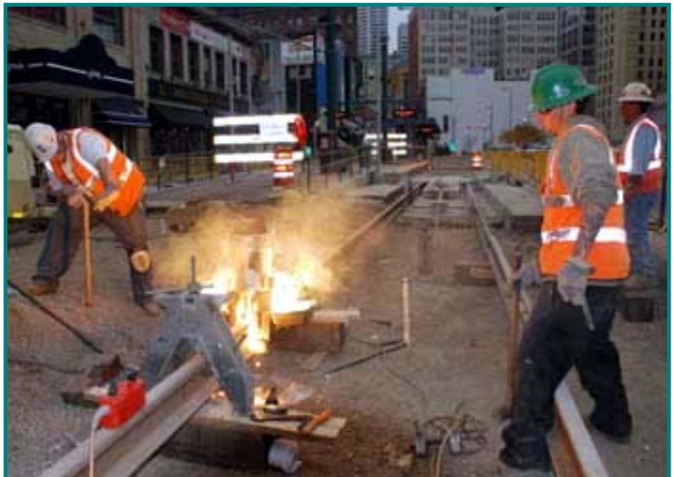
Welders Britton Carpenter and Brian Downey of Chesapeake Thermite Welding finished the final welds in the Hiawatha LRT extension on November 5.
