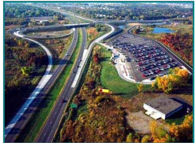
Another 500 parking spaces will be created with the construction of a new parking structure on land adjacent to the current 95th St. park-and-ride lot in Blaine along I-35W.
