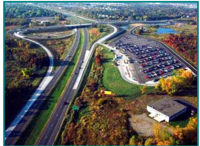
Another 500 parking spaces will be created with the construction of a new parking structure on land adjacent to the current 95th St. park-and-ride lot in Blaine along I-35W.
